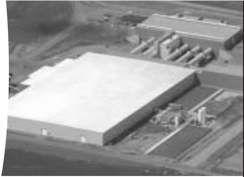
Edmonton Composting Facility
