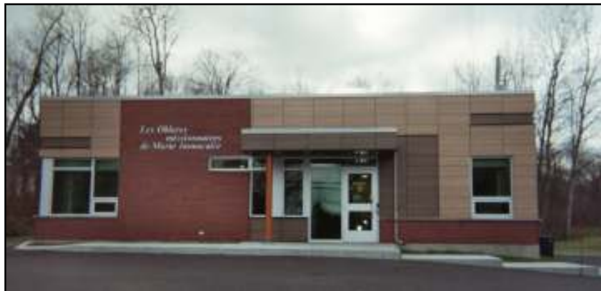
Headquarters – 7625 boulevard Parent, Trois-Rivières.
