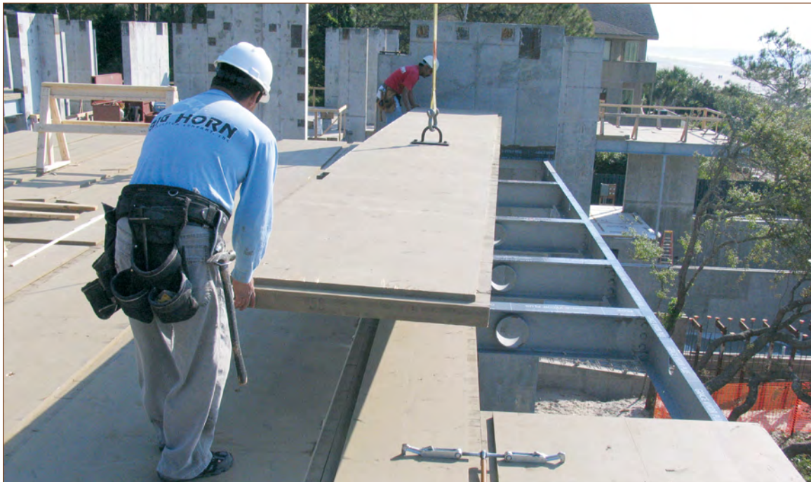
Figure 1 Example of hybrid construction (mass timber slabs with steel structure) (Photo: Binderholz)
