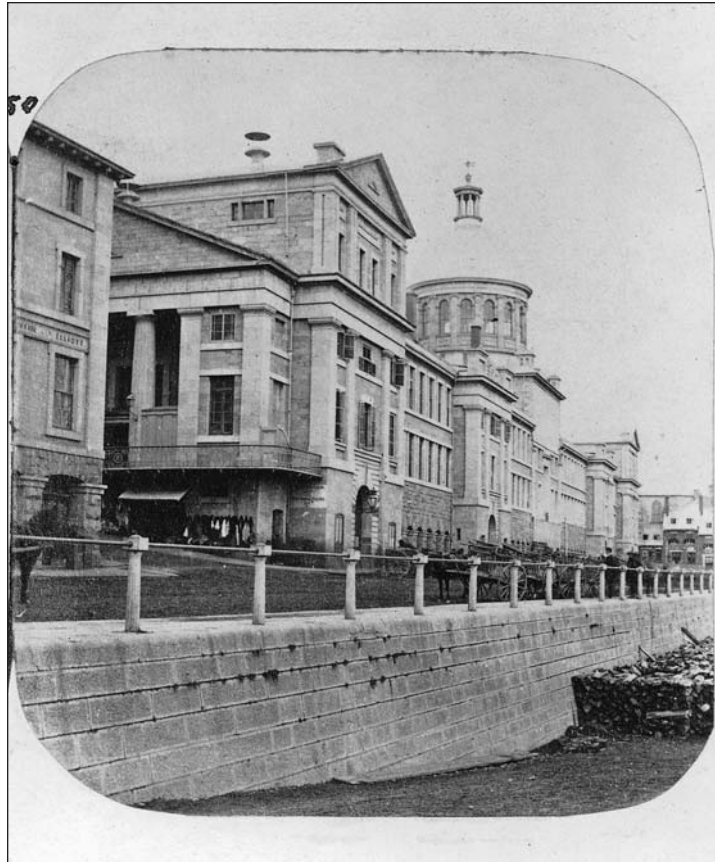
Figure 1.8 Among its accomplishments, the Montreal Harbour Commission raised the level of Commissioners Street and built walls and access ramps, 1859.
