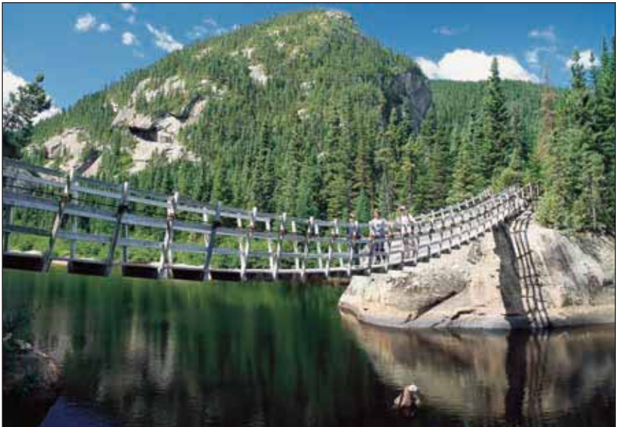
A bridge over Rivière MacDonald leads to the Port-Cartier–Sept-Îles wildlife reserve
