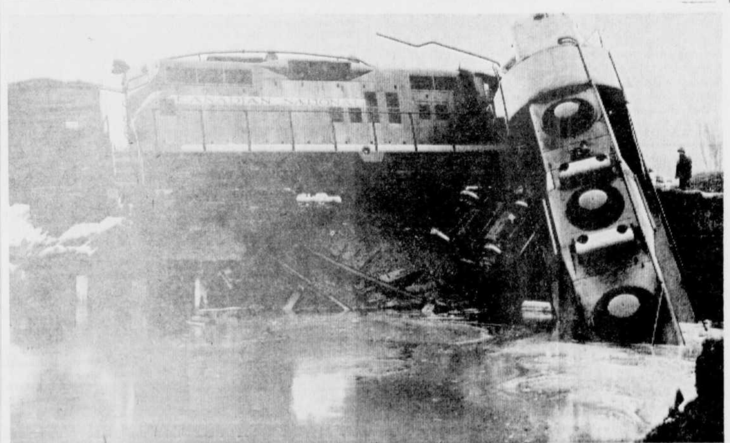
Leading diesel unit of a CNR freight train was thrown into a mud pond when an earth slide caused collapse of tracks near Port Mann, B.C. Boxcar at left bears "Glass" sign. A brakeman was injured but five other crew members were not hurt in the accident which occurred near site of dredging work for a new bridge. (CP Photo)
