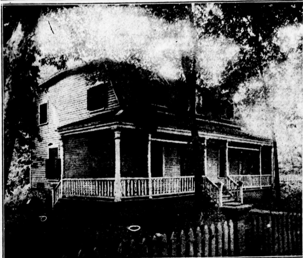
FROM "TOWN HOUSE" TO LAKESHORE SHACK
