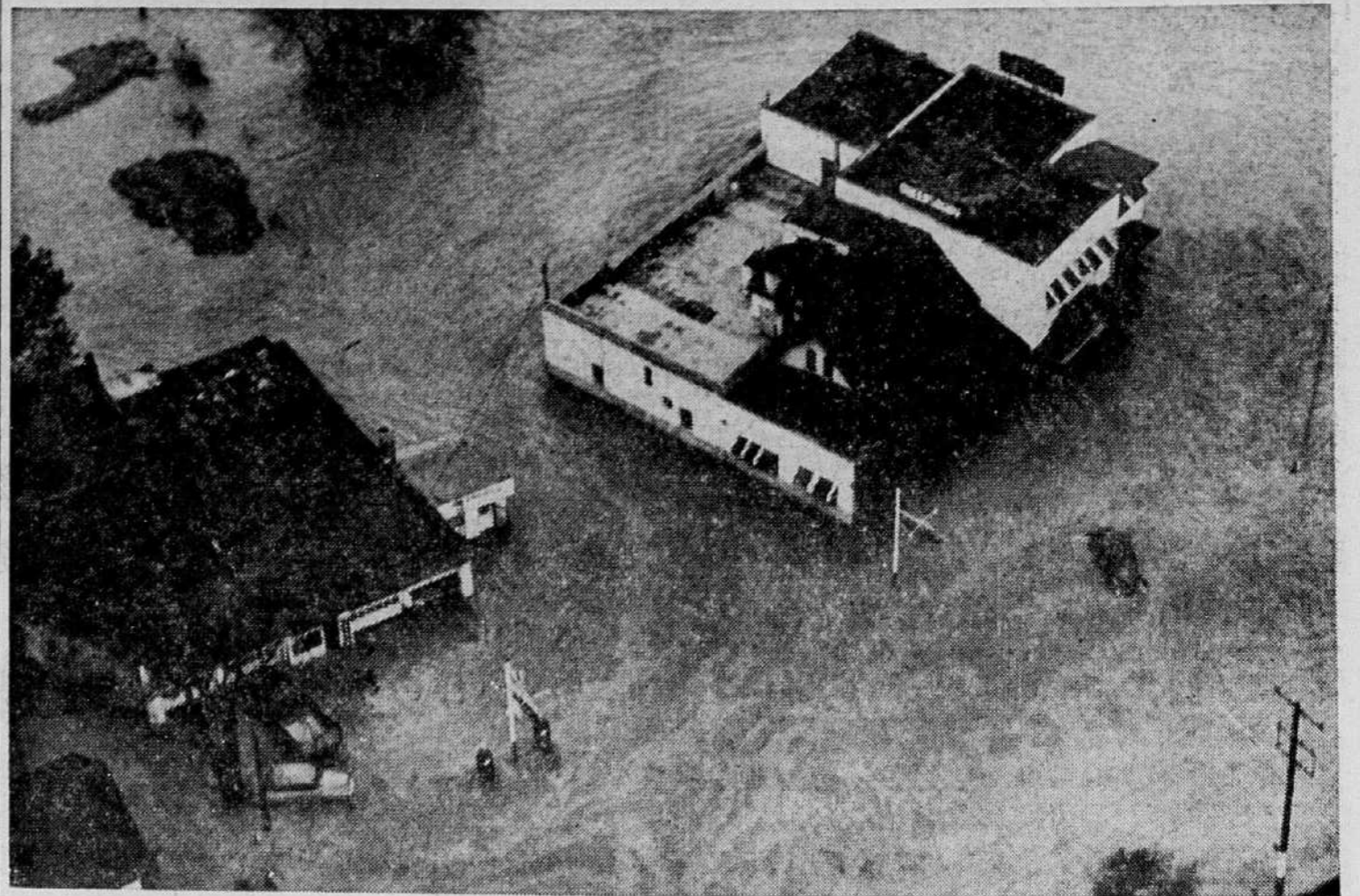
FLOOD CAUSES HAVOC — Hurricane Hazel left a trail of dead, missing and heavy damage when it hit the Toronto area. This hotel and service station in Mount Dennis, a western suburb of Toronto, were partly submerged by flood waters of the Humber river. Motorists had to abandon their cars as the waters drowned their motors. (CP Photo)
