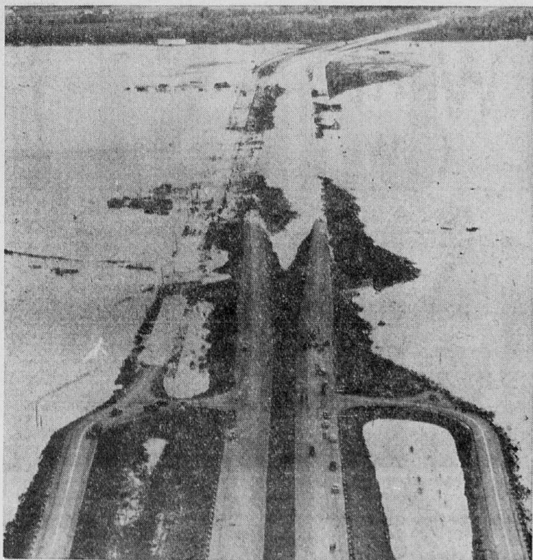
FLOODED HIGHWAY — The Barrie highway, a 50-mile super-highway between Toronto and Barrie, Ont., and the surrounding Holland Marsh are flooded by torrential rains following Hurricane Hazel. The marsh, 30 miles north of Toronto, is a low-lying area of fertile land where hundreds of truck gardeners have farms. Motorists who had to abandon their cars on the highway were taken to the town of Bradford nearby. (CP Photo)
