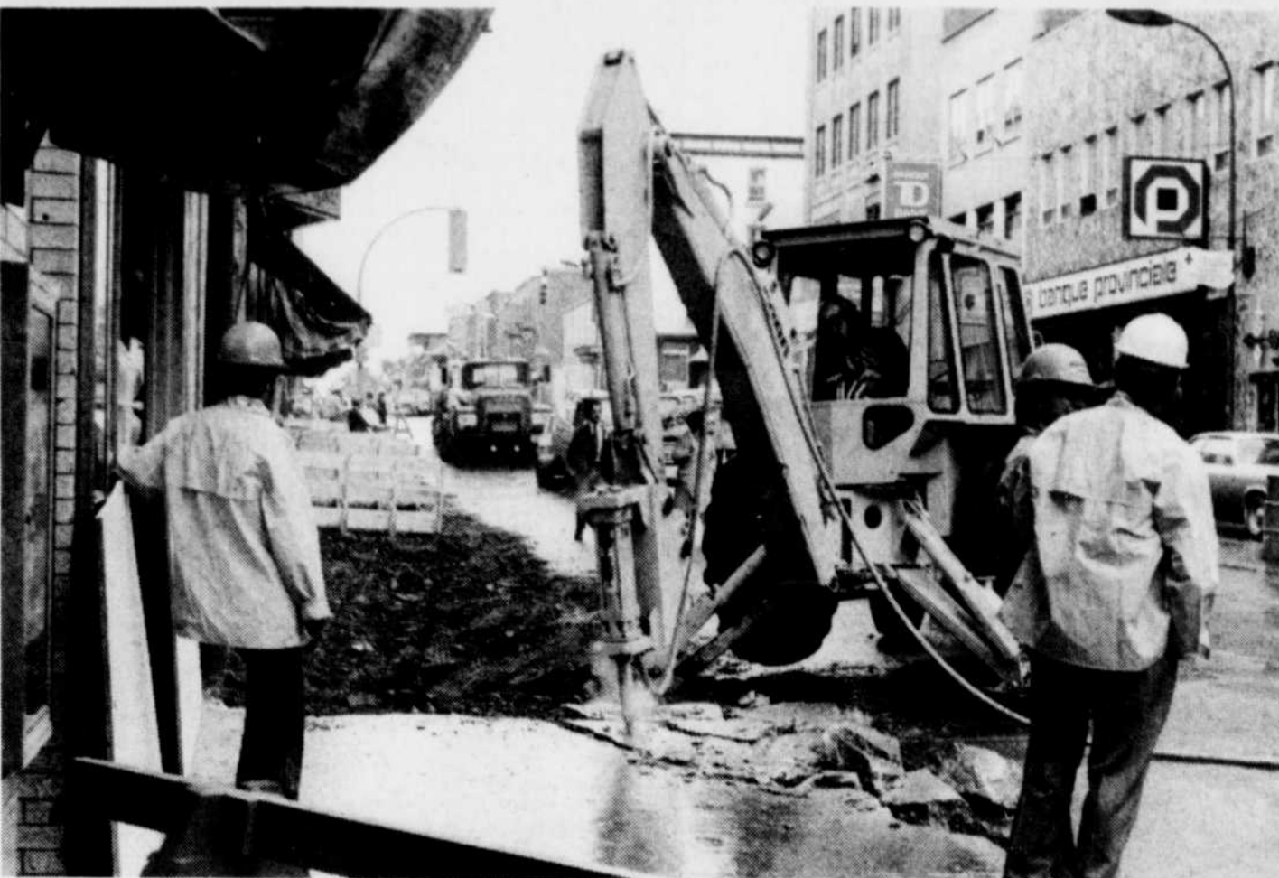
PROJECT BEGINS — Construction on the $2 million downtown revitalization project began Tuesday when workmen moved onto Wellington Street North to demolish the old sidewalks. Traffic
