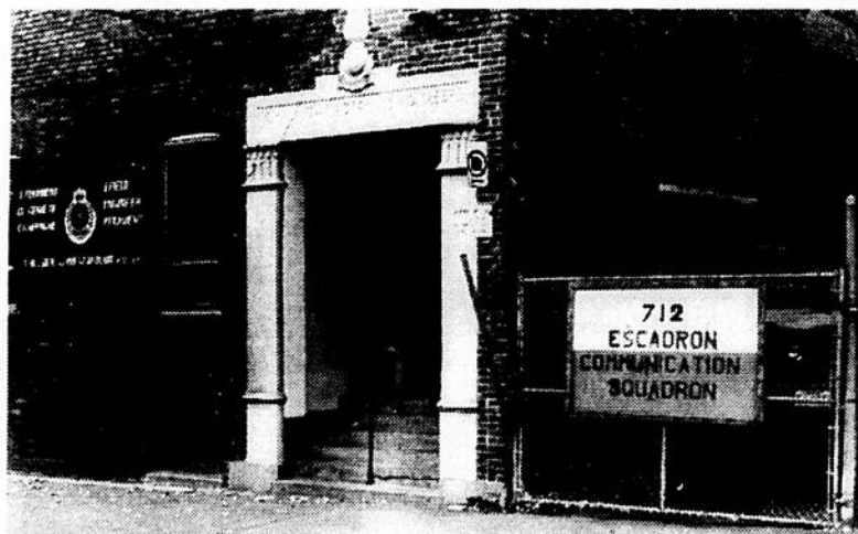
The building housing the 3rd Field Engineer Regiment is decaying, necessitating a move, officers say.
