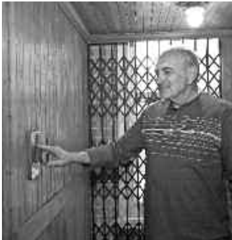
Irving Kaplan stands in the elevator in his heritage home at 413 Roslyn Ave. The solid oak elevator has the original brass controls and scissor doors.
