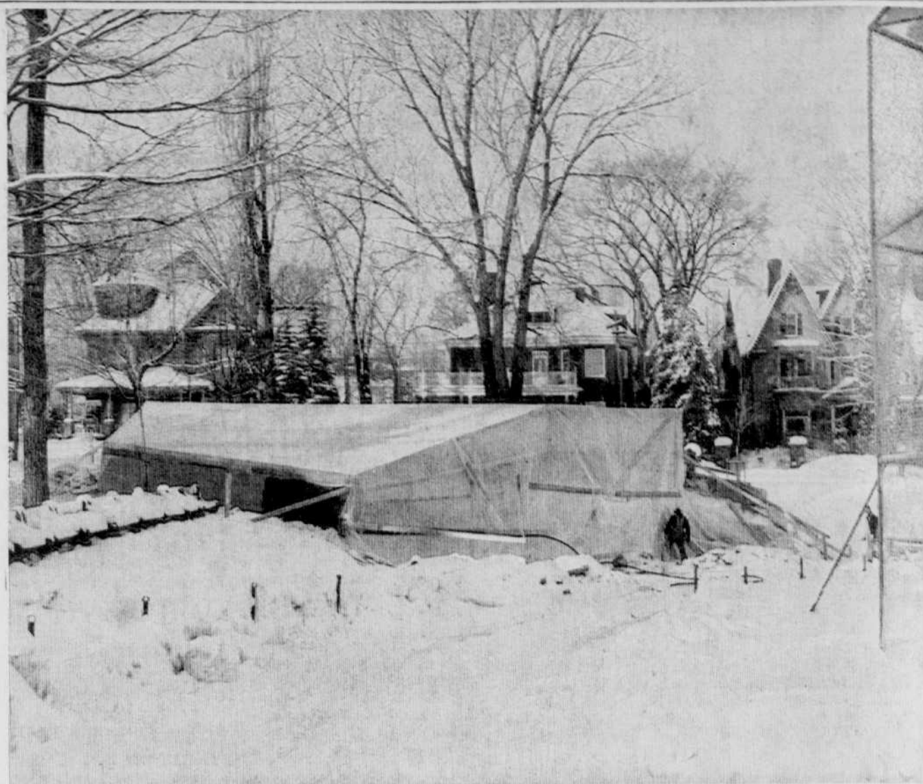
AT PARADE GROUNDS — Work started on the Parade Grounds washrooms January 10, and should be completed by the end of February, according to Paul Talbot, the general contractor in charge of the job. The size of the structure is to be about 1,000 square feet and is being built at a cost of close to $15,000 said Mr. Talbot. The site of the structure is the Parade Grounds on Moore Street and Queen Boulevard. (Record photo by Gerry Lemay)
