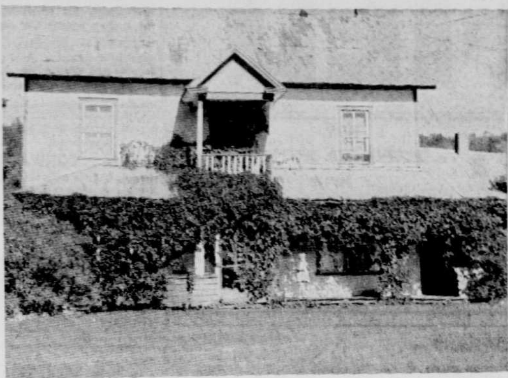
HOME FOR SENIOR CITIZENS — Pictured above is the lovely old building at Kinnear's Mills, formerly the manse of Candlish United Church, which has been purchased by an interested group for conversion to a home for elderly people in the Megantic county area. A campaign is under way to raise funds for extensive renovations to the well constructed building and for the addition of a 27 by 60 foot wing on the north-west side. A similar wing could be erected on the south-east should conditions warrant it.
