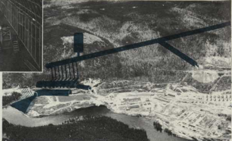
A 7.6-mile tunnel, 35 feet in diameter and excavated in solid rock, will bring the waters of Lac Cassé 875 feet downward to the underground generating station
