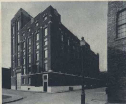
Vallée Stn. 75,000 KVA — 60/4KV
