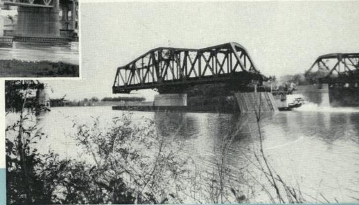
Below: SWING BRIDGE at Kildonan, Manitoba carrying double tracks of the C. P. Railway over the Red River.
