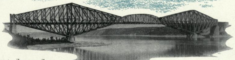
1912-1917 The Quebec Bridge—Largest railway cantilever bridge in the world, spanning the St. Lawrence River near Quebec City. Length between main piers: 1800 feet. Total weight of steel: 65,000 tons.
