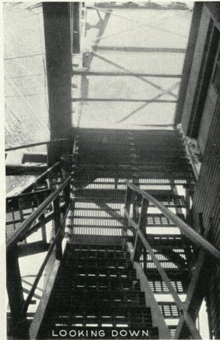
Above: Stairs for service and emergency use equipped with "M & M" platforms and treads.
