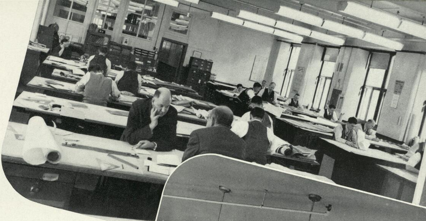
Above: Part of the plate and boiler design department.
