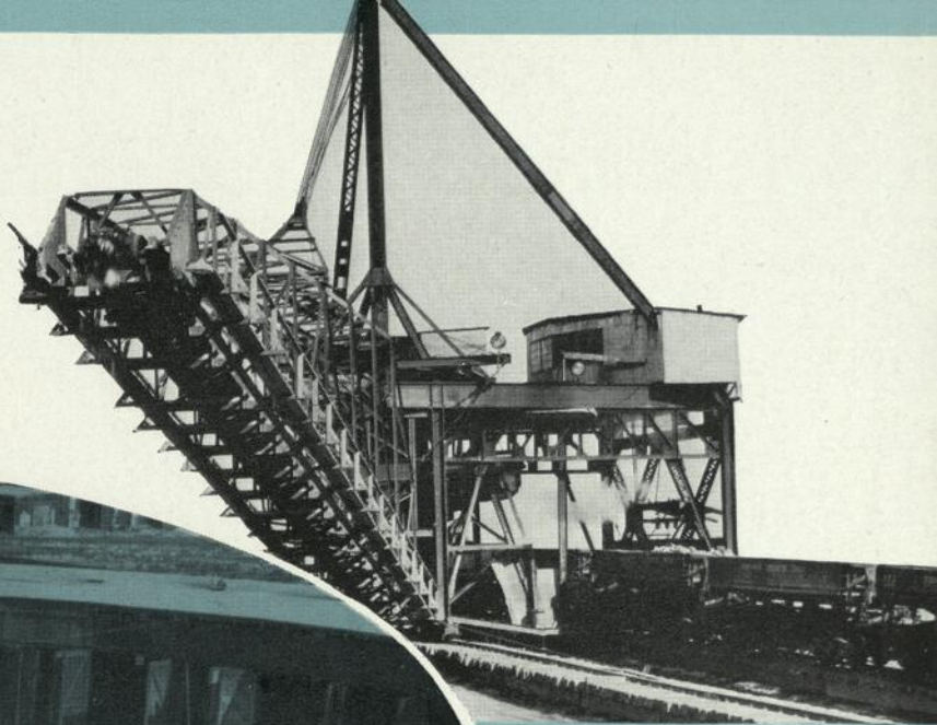
Right: Special equipment for laying rip-rap to prevent erosion of the sides of a canal.
