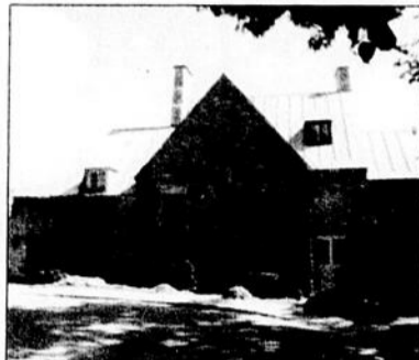
TRADITIONAL STONE COTTAGE WESTMOUNT $3,150,000
