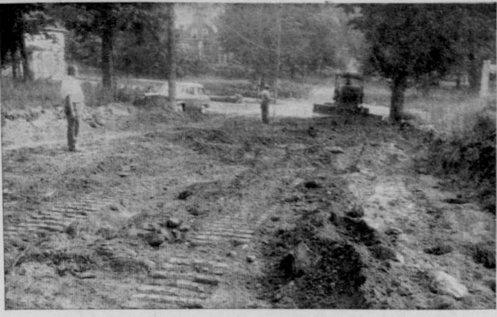
WIDENING — Photo shows widening and repaving of Waterloo's Western Avenue.
