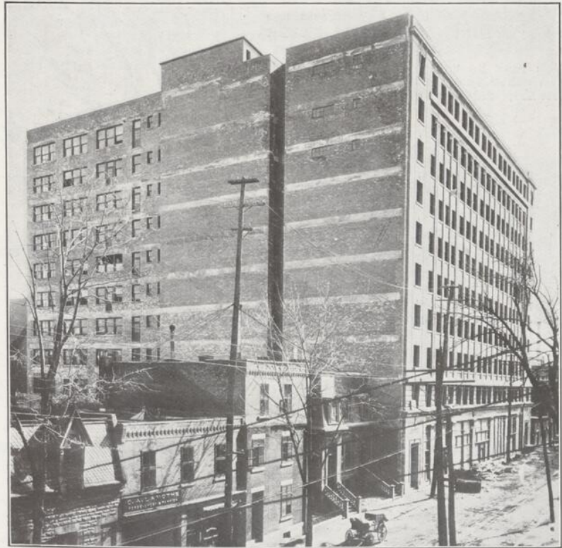
MODERN MONTREAL—The Sommer building now rapidly approaching completion on Ontario street west in close proximity to St. Catherine and Bleury streets, two of the city's great business arteries.
