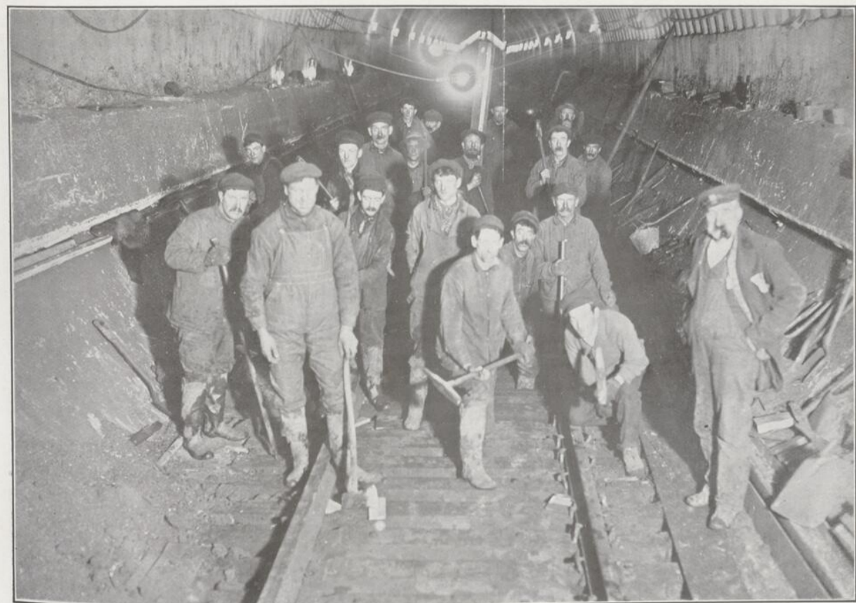
A TRACK REPAIRING CREW AT WORK IN THE ST. CLAIR TUNNEL—This tunnel extends under the River St. Clair from Sarnia, on the Canadian side, to Port Huron, on the American side. It is considerably over a mile in length (6,025 feet) and through it trains of the Grand Trunk Railway pass on their way from Montreal to Chicago and vice versa. With its approaches the tunnel is over two miles in length. Formerly trains were hauled through the tunnel by powerful steam locomotives, but the deadly fumes and gases generated by these made it necessary to install electric locomotives. In the above picture a repairing crew is laying new rails in the centre of the tunnel. This work can only be done at certain hours of the night when traffic is light.
