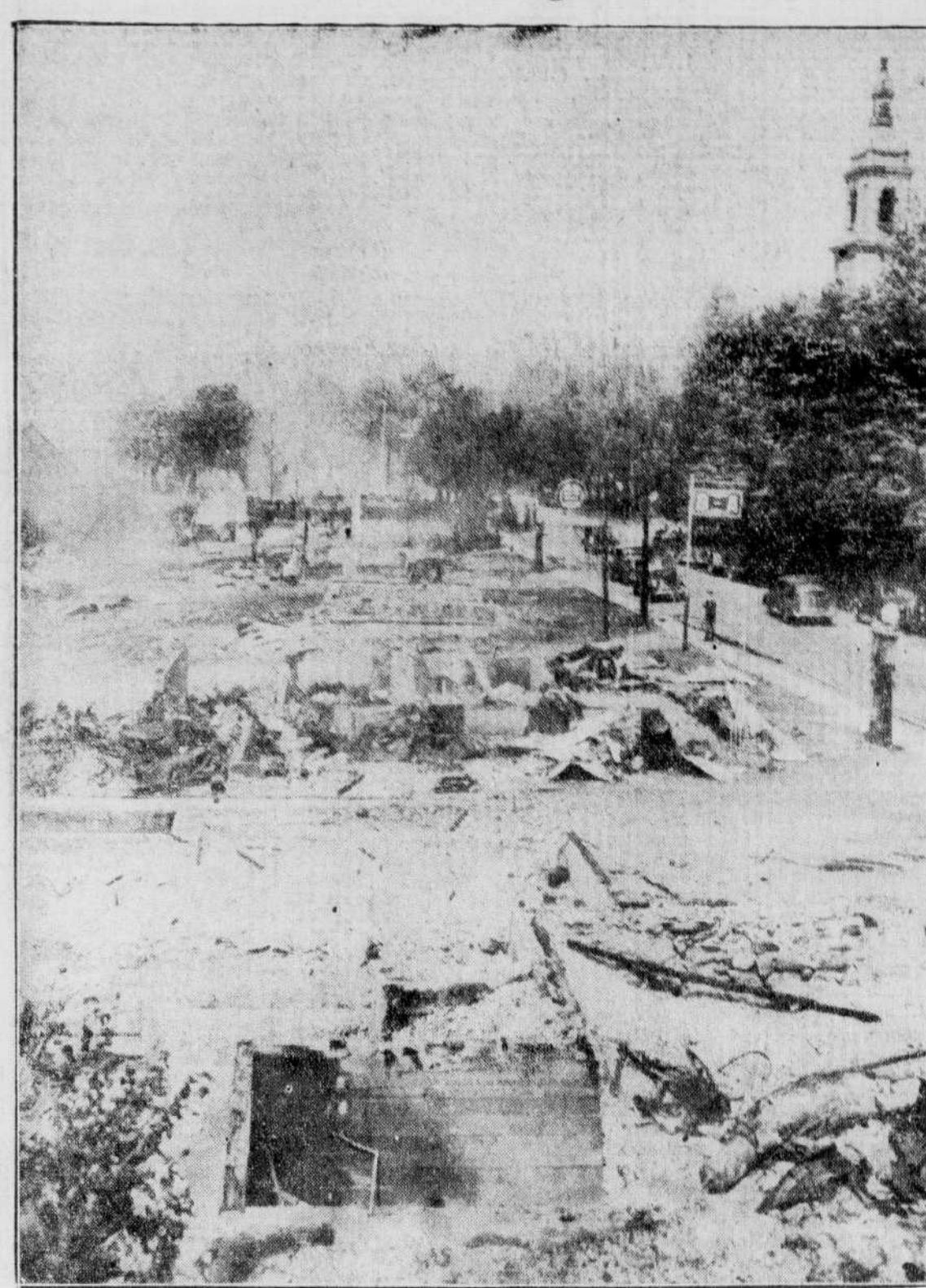
A general view of the site where six buildings were burned to the ground in the Katevale conflagration on Saturday morning, taken some hours after the blaze had died down. While the fire raged, it was impossible to take any photographs due to the tremendous amount of smoke and heat waves which registered only a grey mass on the film. Apart from a few household belongings and a number of head of cattle, the buildings were a complete loss.
