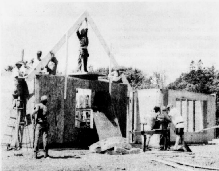
The construction crew usually got started on Sunday mornings.
