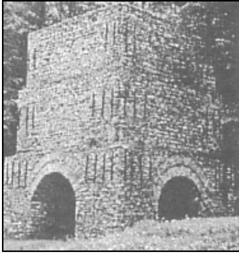
Figure 2.57: Ruins of an 18th century blast furnace.
