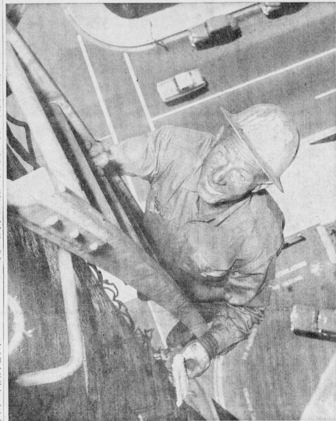
HIGH MAN ON STACK — Way up there went a newspaper photographer in Vancouver to get this picture of steeplejack Frank Specht, repainting the 195-foot smoke stack above Vancouver General Hospital's power plant. (CP Photo)
