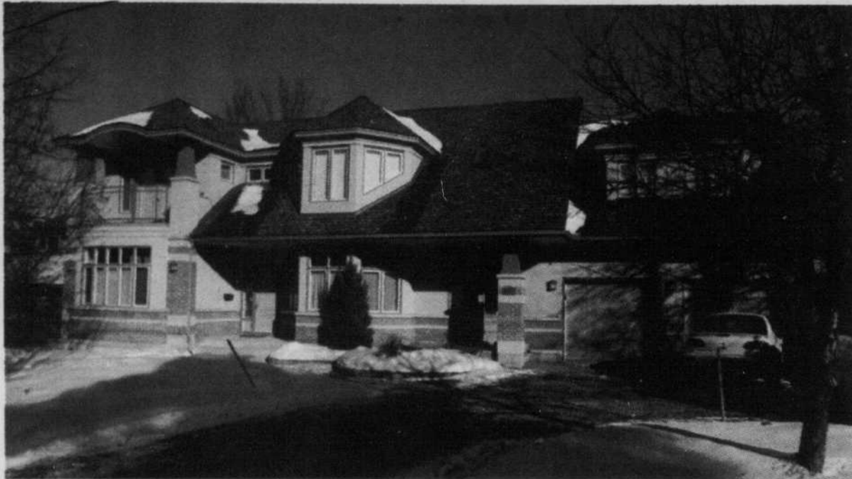
Large overhangs on the front of Roy Nandram's house effectively shade windows in the summer, keeping inside spaces cool.
