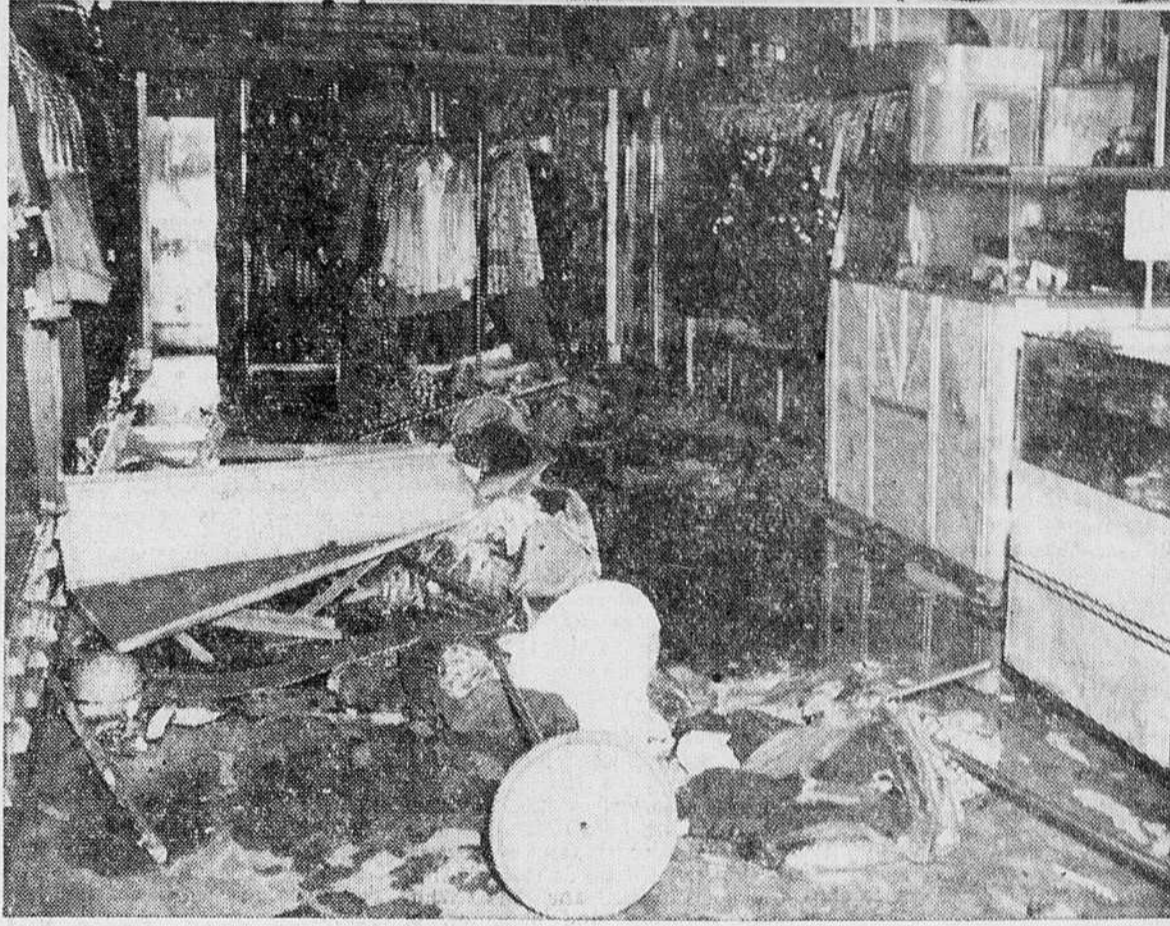
DEPARTMENT STORE FIRE: The top photo shows the front of the J. A. Savard store which suffered heavy loss in yesterday's noon fire. Firemen are shown in action as the heavy smoke pours from the interior of the store. Three firemen were overcome by smoke and required hospital treatment. The bottom photo shows the heavy damage which was inflicted on the ladies' department of the store. The basement was completely burned out and all the stock there in ruins. Damage to building and stock is estimated at more than $75,000. J. A. Savard Limited hopes to have the men's department open in five or six days but the ladies' section may not be in operation again for two weeks. (Record photos by Gerry Lemay).
