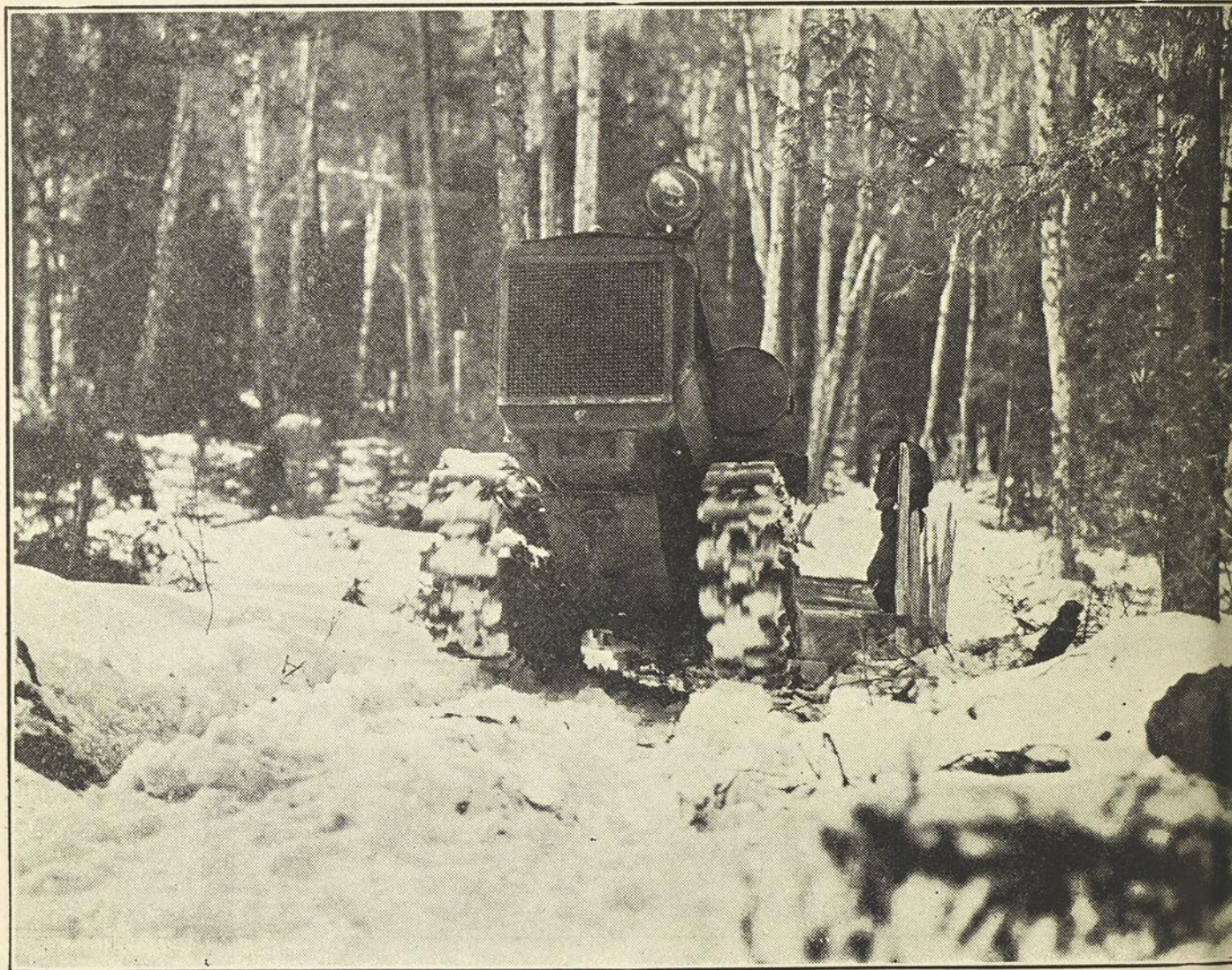
Provincial Pulp and Paper Co. Port Arthur, Canada. "Caterpillar" Thirty coming up with empty sleigh to be loaded with pulp wood. Thirty actually runs into the strip roads and loads up. Total cost everything figured on 4\frac{1}{2} mile haul $1.45 a cord.
