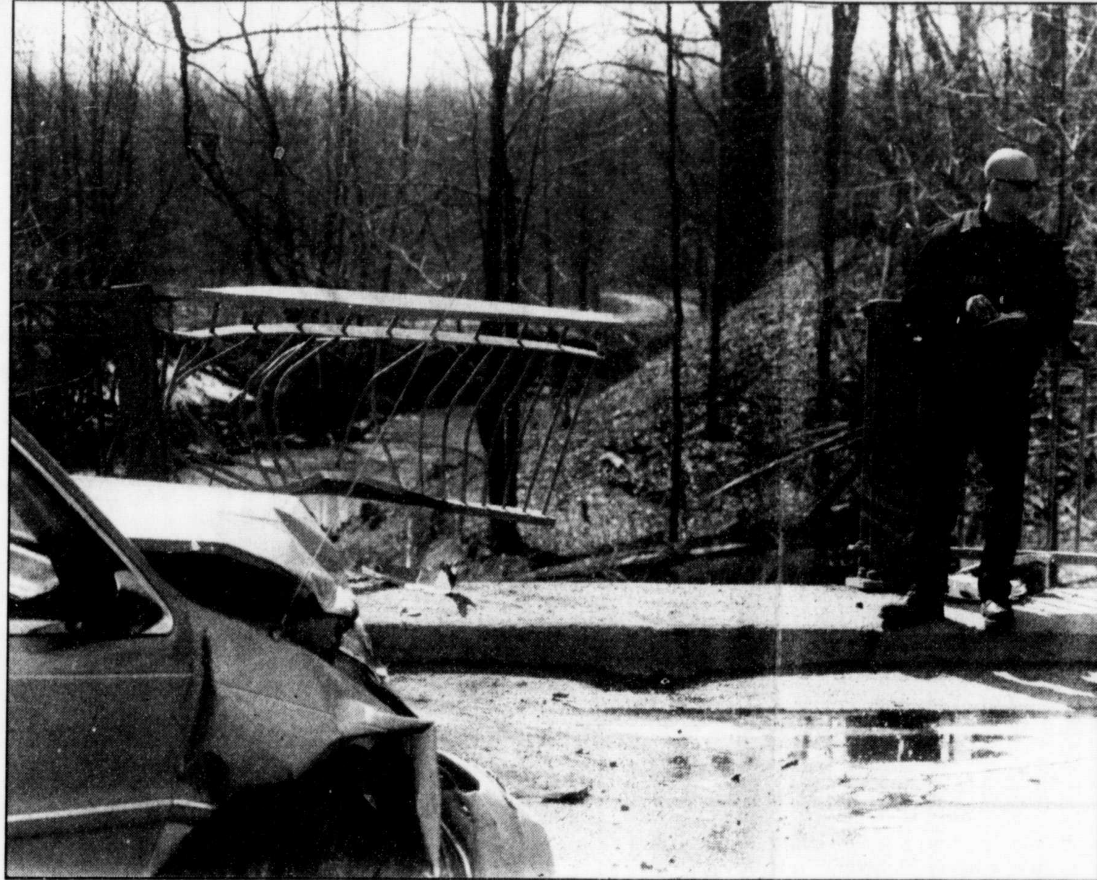
A BRIDGE TOO CLOSE: The driver escaped serious injury when her car (foreground) hit the bridge on Hwy. 148 near Breckenridge. A MRC des Collines police officer is seen here investigating the accident shortly after it happened Friday afternoon.
