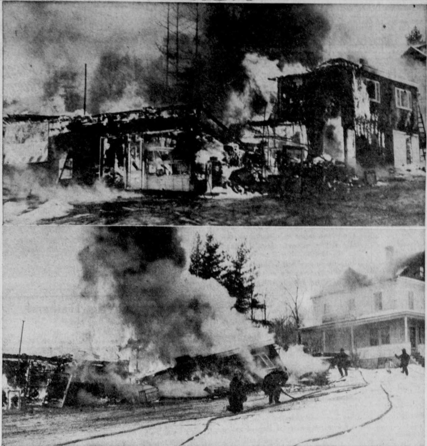
North Ward Fire — Sherbrooke firemen from stations Nos. 1 and 5 managed to save the house of J. R. Latulippe, at 3335 King St. West, yesterday afternoon despite high winds which blew flames from an adjoining foodstuff warehouse, owned by Mr. Latulippe, that was completely destroyed. In the top picture, the warehouse is seen just before it collapsed, while below firemen roll out their lines to spray Mr. Latulippe's home.
