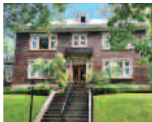
AV. MAPLEWOOD, OUTREMONT $2,275,000
