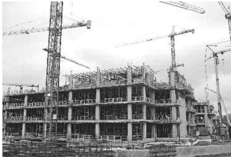
Westmount can still be seen from the NDG side of the under-construction super hospital site, but that will soon change as the building is quickly climbing skyward.
