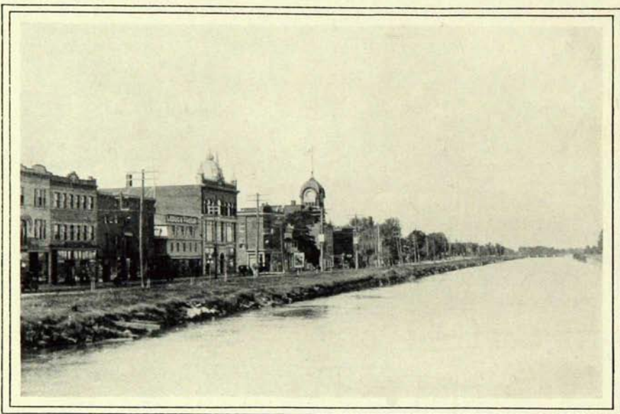
A section of Valleyfield and Old Beauharnois Canal, Highway No. 3
