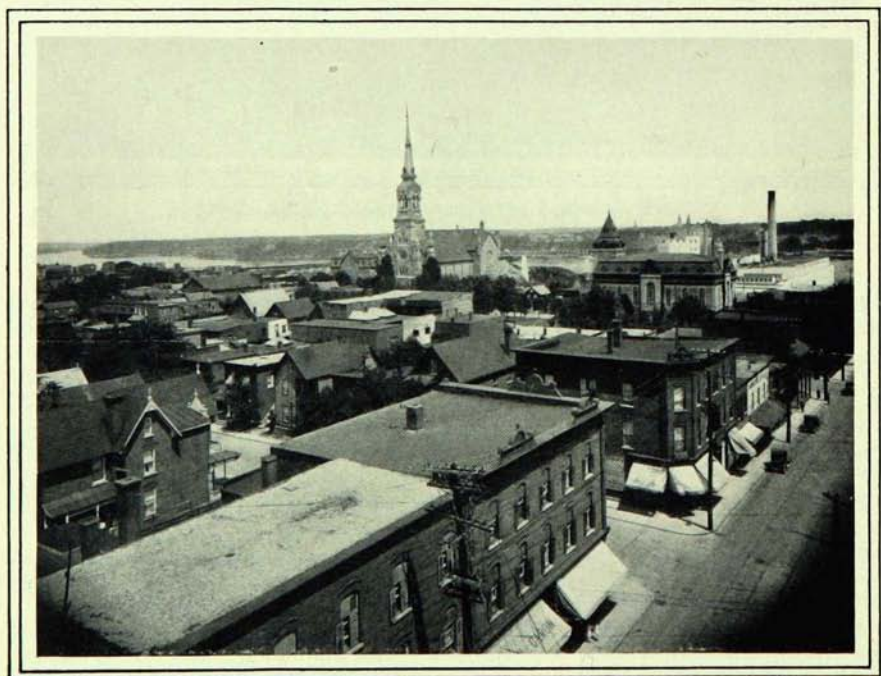
A section of Hull, on Highway No. 8
