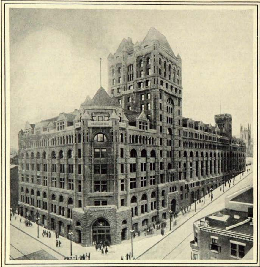
Windsor Station, Canadian Pacific Railway, Montreal
