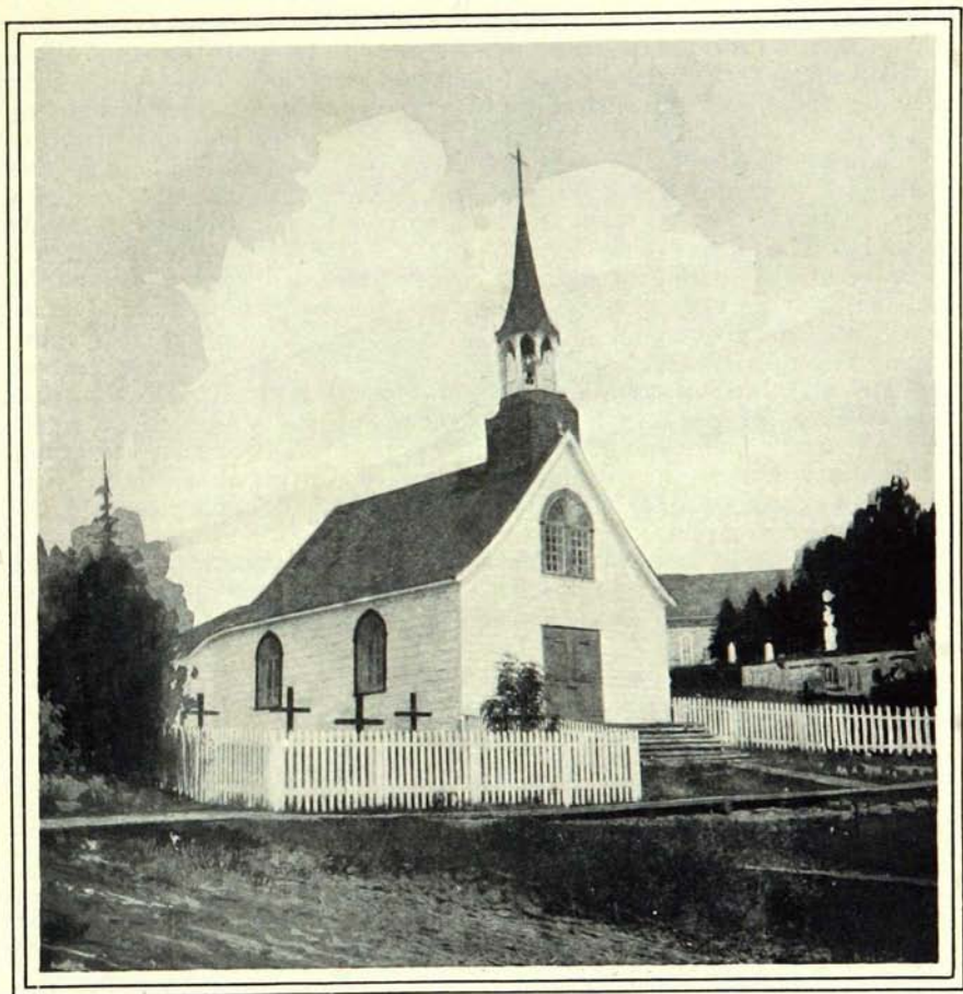
The Old Chapel, Tadoussac, Highway No. 15A
