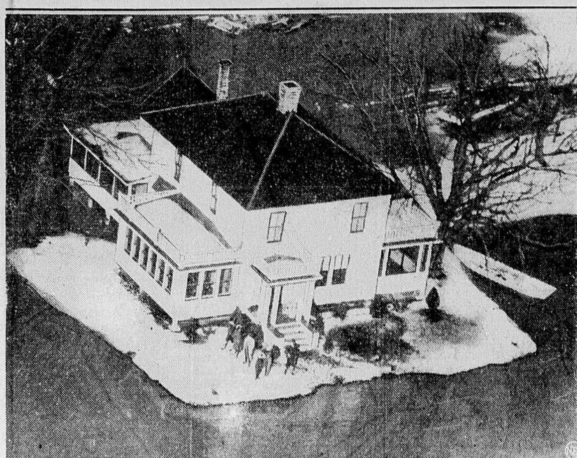
Most colonists at the Dress, Ark., farm resettlement project fled when the St. Francis River flooded their homes. The few hardy souls who defied the overflow are seen in this air view clustered about the porch of one of the buildings on higher ground. A boat for flight in extreme emergency is conveniently moored at right.
