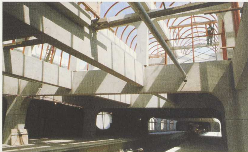
Angrignon station under construction. (STM archives)
