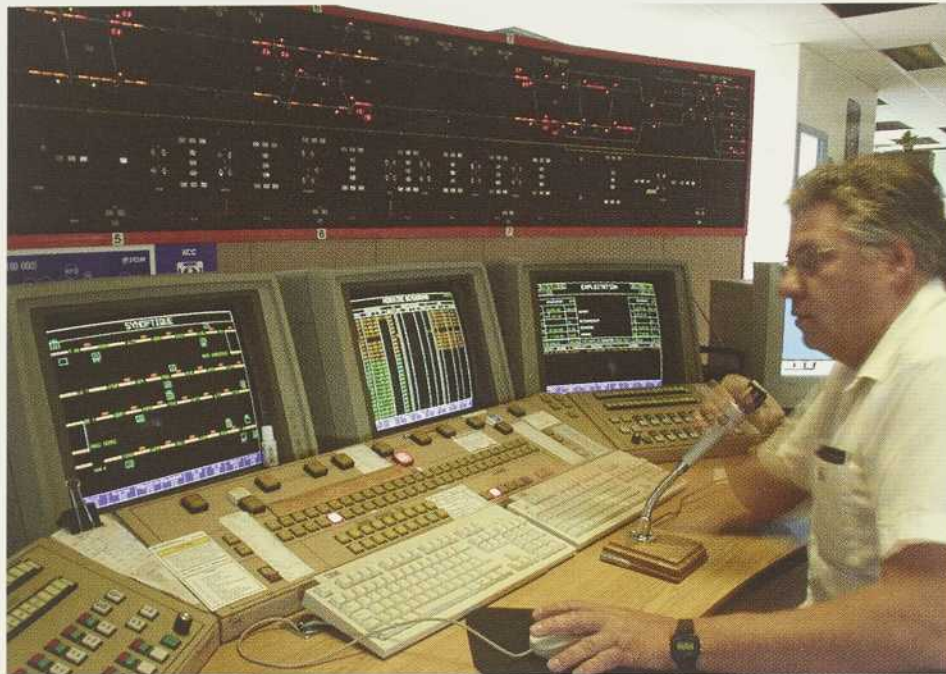
PCC traffic controller before a visual display board pinpointing the flow of trains. (Michel E. Tremblay - STM)
