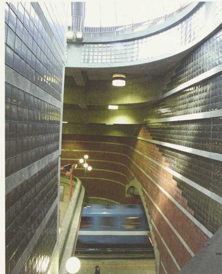
Natural light shaft at Outremont station. (Michel E. Tremblay - STM)
