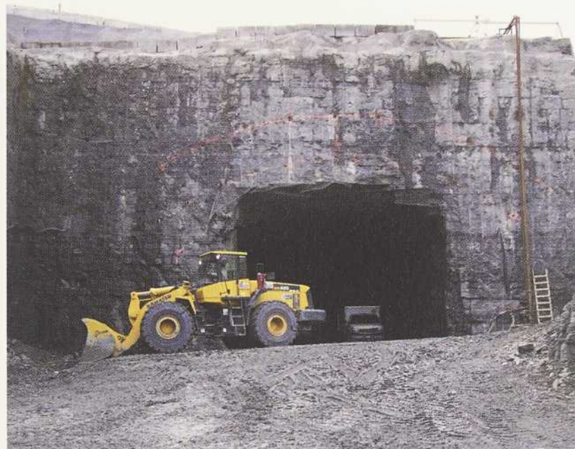
De la Concorde station under construction. (Agence métropolitaine de transport)
