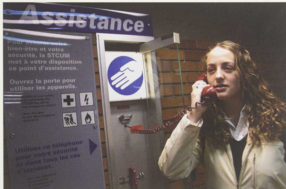
Each train platform holds at least one emergency telephone linked directly to the Control Centre. (Michel E. Tremblay - STM)
