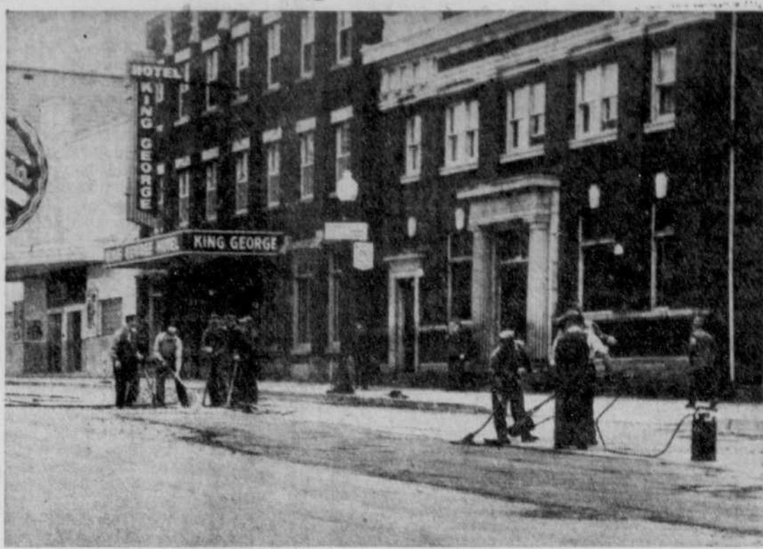
Workmen are busy repairing Sherbrooke's streets these days and they've got a lot of work ahead of them. City streets suffered severely during the winter and spring months. In this picture a crew is shown repairing a stretch of King St., west. (Record Photo by Gerry Lemay)
