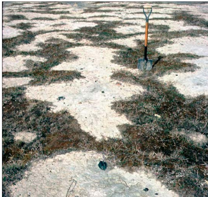
FIGURE 5.33: MUDBOILS EXTENDING DOWN A SLOPE.
