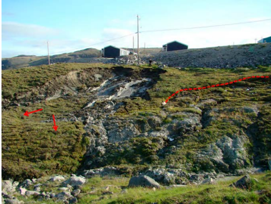
FIGURE 5.43: ACTIVE LAYER STRIKE-SLIP SLIDE AT SALLUIT ON AUGUST 22, 2010. WE SEE THE STRIKE-SLIP FAULT IN THE ACTIVE LAYER AND THE NEWLY EXPOSED ICE-RICH PERMAFROST. THE PLANT COVER AND ACTIVE LAYER SLID TO THE BOTTOM OF THE SLOPE. AT THE RIGHT, THE DOTTED LINE INDICATES A SIMILAR STRIKE-SLIP FAULT SLIDE THAT OCCURRED IN 2005.
