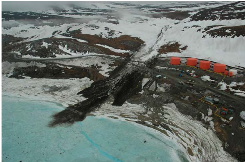
FIGURE 5.44: SLUSH AVALANCHE THAT TOOK OUT A PORTION OF THE BAIE DÉCEPTION ROAD ON MAY 15, 2005.
