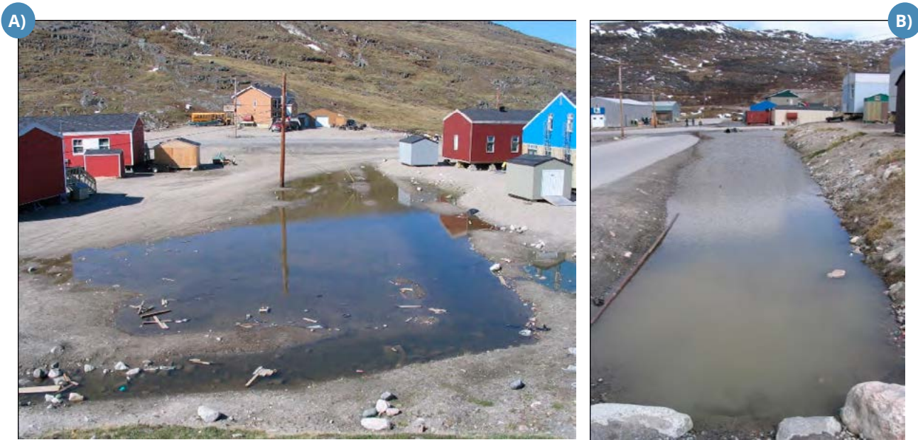
FIGURE 5.91: MAJOR WATER ACCUMULATION A) NEXT TO FILL AND B) IN A DRAINAGE DITCH (SOURCE: E. L'HÉRAULT, CEN, 2008).
