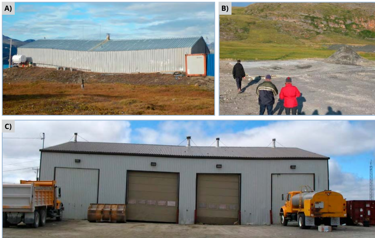
FIGURE 5.53: SERIOUS DEFORMATION AND DAMAGE CAUSED TO SLAB-ON-GRADE FOUNDATIONS BY COMPACTION AND CONSOLIDATION AT TIME OF THAWING OF ICE-RICH PERMAFROST. A) HEATED WAREHOUSE AT PANGNIRTUNG, NUNAVUT. B) SLAB OF FORMER FIREHALL IN THE MUNICIPALITY OF SALLUIT, NUNAVIK. C) FORMER MUNICIPAL GARAGE OF THE MUNICIPALITY OF TASIUJAQ, NUNAVIK.
