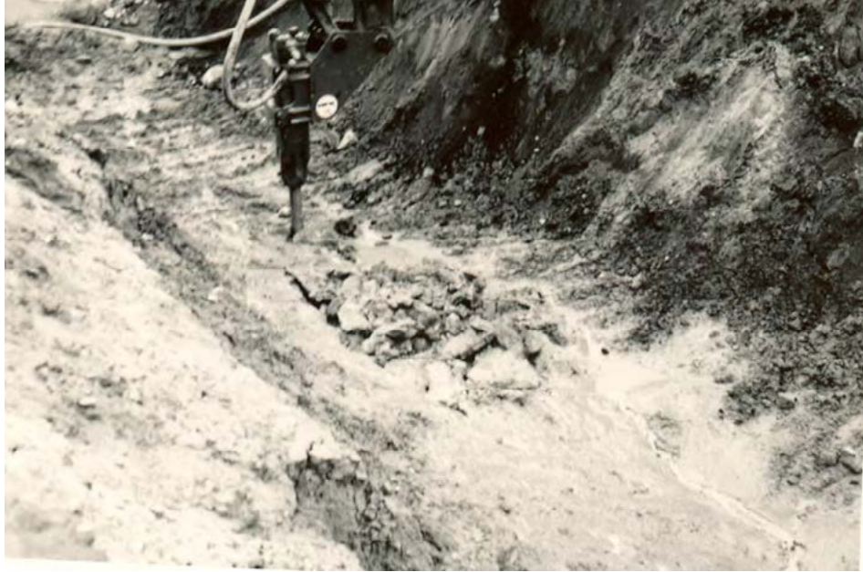
FIGURE 5.18: PERCUSSION HAMMER EXCAVATING PERMAFROST IN TILL AT KANGIQSUALUJJUAQ.
