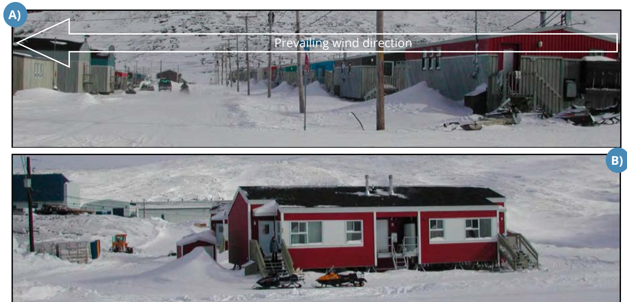
FIGURE 5.88: A) HOMES WITH THE LONG AXIS PERPENDICULAR TO THE PREVAILING WINDS. B) HOME WITH THE LONG AXIS PARALLEL TO THE PREVAILING WINDS (FROM ALLARD ET AL., 2010).
