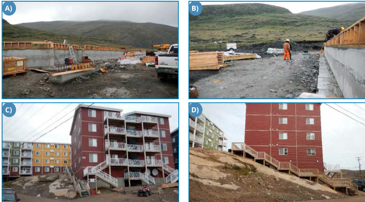
FIGURE 5.70: A) AND B) FOUNDATION WALL ON A CONTINUOUS FOOTING RESTING ON A GRADED ROCKY SUBSTRATE AT KANGIQSUJUAQ, NUNAVIK. C) AND D) FOUNDATION WALL ON A CONTINUOUS FOOTING RESTING ON AN SLOPED ROCKY AT IQALUIT, NUNAVUT.
