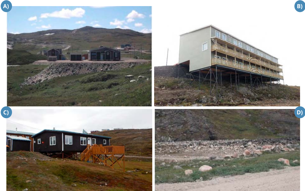
FIGURE 5.92: A) VERY THICK GRANULAR FILL ON SLOPED LAND AT SALLUIT, NUNAVIK. B) AND C) FOUNDATION SYSTEM ADAPTED TO THE TOPOGRAPHY, RESTING DIRECTLY ON ROCK AT IQALUIT, NUNAVUT. D) CRUSHER REJECTS USABLE FOR CONSTRUCTION OF GRANULAR INVERTS (SOURCE: N. JOURNEAUX).
