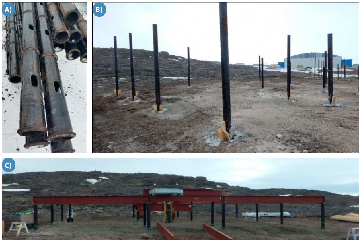
FIGURE 5.77: A) PILES TO WHICH STEEL COLLARS HAVE BEEN WELDED AND IN WHICH HOLES HAVE BEEN DRILLED TO INCREASE BEARING CAPACITY (SOURCE: G. ROBICHAUD, 2015). POINT-BEARING PILES USED FOR AN SHQ PROTOTYPE HOUSE FOUNDATION AT QUAQTAQ DURING B) SLURRY PLACEMENT AND C) ONCE CUT LEVEL WITH THE RIBBON JOIST ATTACHED (SOURCE: E. L'HÉRAULT, CEN, 2015).
