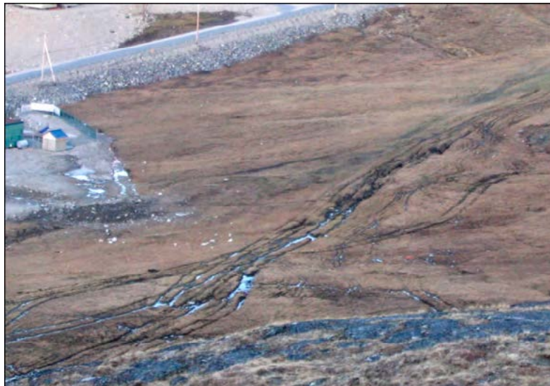
FIGURE 5.20: RUTTING IN ACTIVE LAYER CLAY MARINE SEDIMENTS CAUSED BY MACHINERY AND AFFECTED BY THERMAL EROSION.
