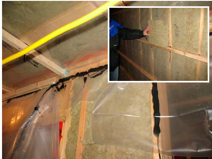
FIGURE 3.6: WATER VAPOUR SYSTEM ON INTERIOR WALL FACE. SOURCE : SHQ
