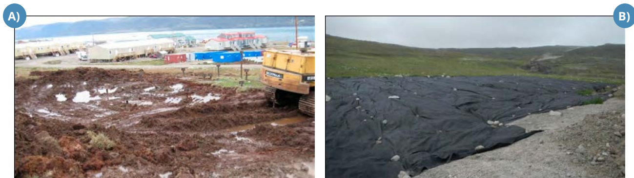
FIGURE 5.85: A) DISTURBANCE OF LAND DURING INSTALLATION OF A PILE FOUNDATION AT PANGNIRTUNG, NUNAVUT (SOURCE: E. L'HÉRAULT, CEN, 2010). B) PLACEMENT OF GEOTEXTILE OVER NATURAL SOIL TO AVOID MIGRATION AND MIXING OF MATERIALS IN SITU WITH THOSE MAKING UP THE GRANULAR FILL, AT SALLUIT, NUNAVIK.
