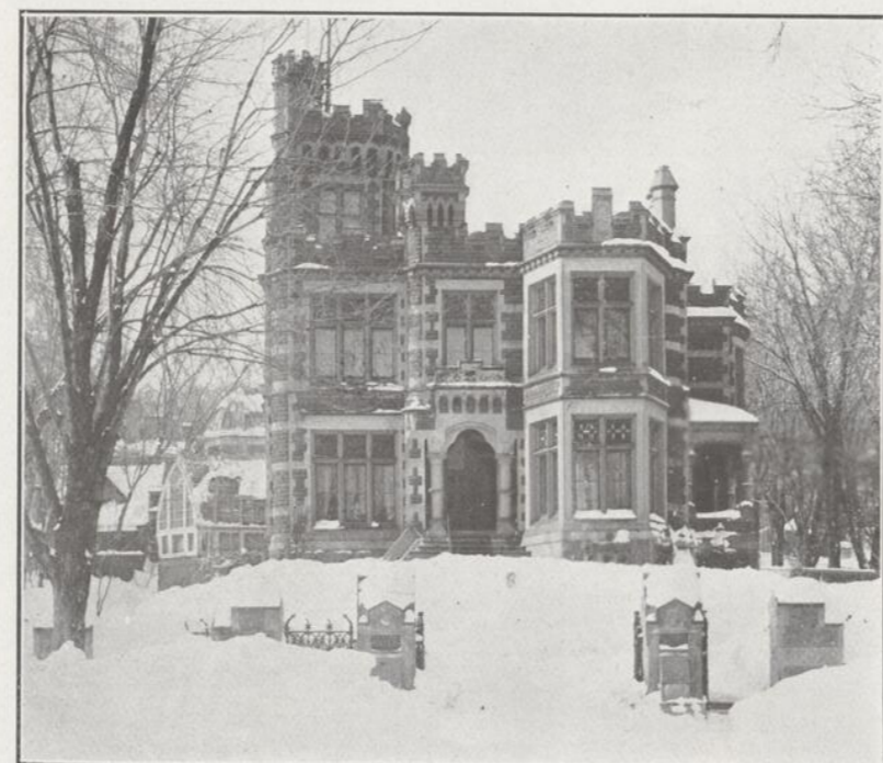
THE STATELY HOMES OF CANADA—"Rokeyby," the charming town residence of Mrs. A. F. Gault, Sherbrooke street West, Montreal.
