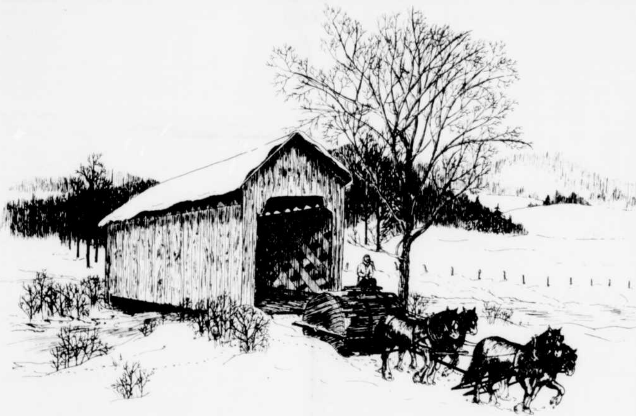
Snow removal during the days of the horse and sleigh was a difficult operation. The snowroller, pictured above, was more common in villages, due to its size, and often two teams of horses were used to pull it.
