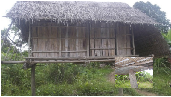
Legkew ; posts are fitted with round slab to protect rodent to get into the storagehut.
