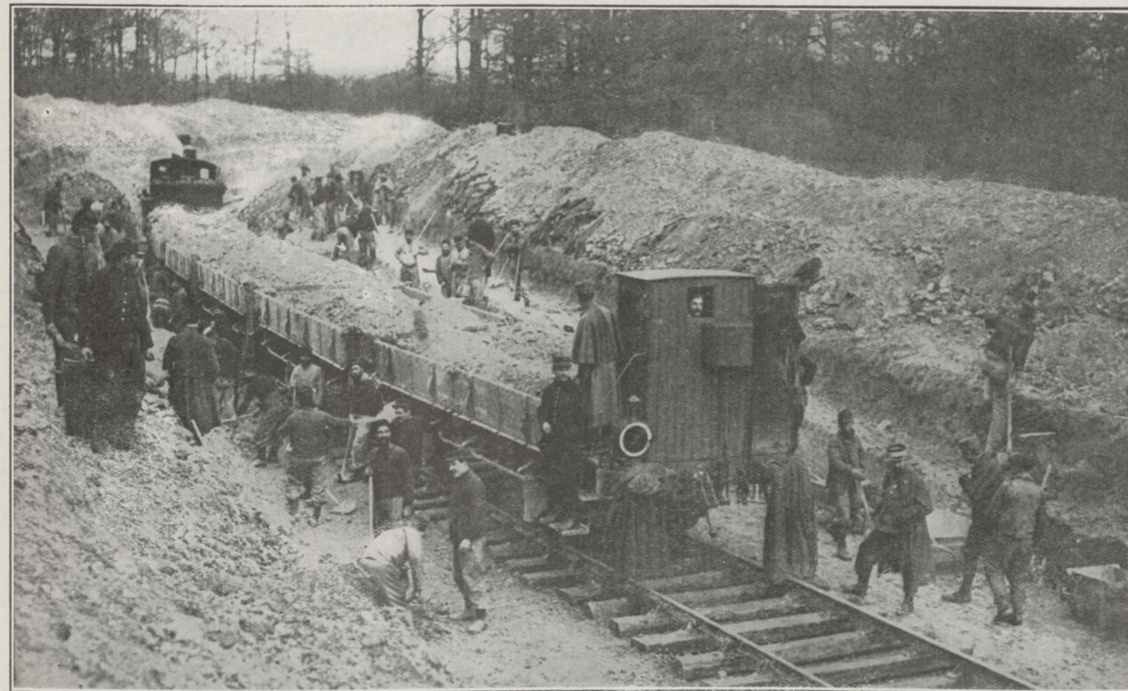
BUILDING A STRATEGICAL RAILWAY ON HISTORIC GROUND.—This road, over which thousands of French troops have been transported to the front, was completed in three weeks. That portion of it shown in the above illustration passes through the woods of Malmaison, the home of the Empress Josephine after Napoleon had divorced her.
