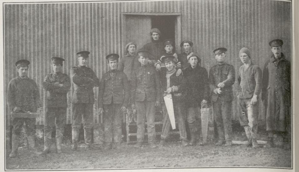
CANADIAN HUT BUILDERS AT SALISBURY PLAIN—A detachment from the 1st Montreal Regiment which is assisting in the task of constructing the winter homes of the Canadian boys at Larkhill Camp. Each hut is 20 ft. wide by 60 ft. long and accommodates 42 non-commissioned officers and men.
