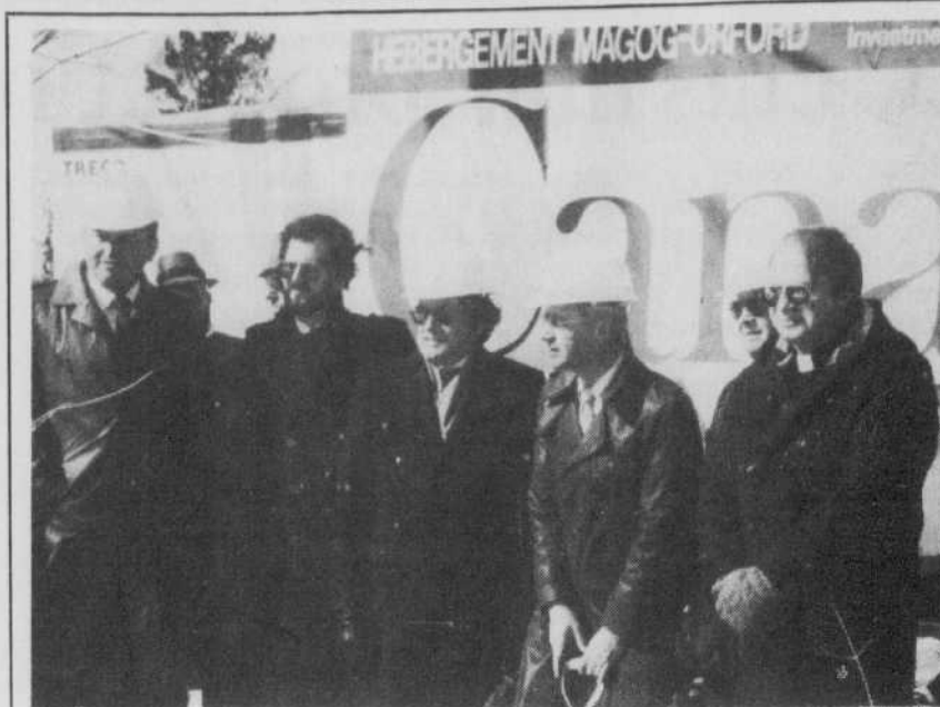
Attending the ground-breaking ceremony in Magog March 17 marking the construction of 26 apartments for senior citizens was (left to right) Gary Longchamps, general contractor; Bernard Wirich, manager, CMHC; André Bachand, Brome-Missisquoi MP; Paul-René Gilbert, president, Hébergement Magog-Orford; and Rev. L. Ross, Magog Anglican Church.
