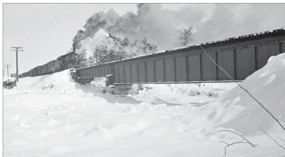
Bromptonville CNR bridge with train, 1935
