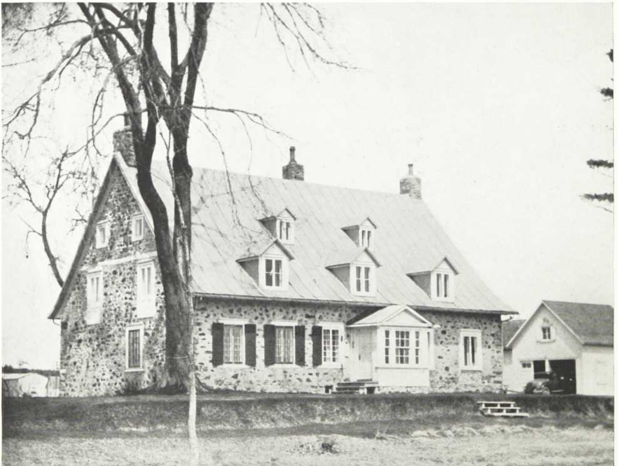
THE SOUTH SIDE AFTER RESTORATION
