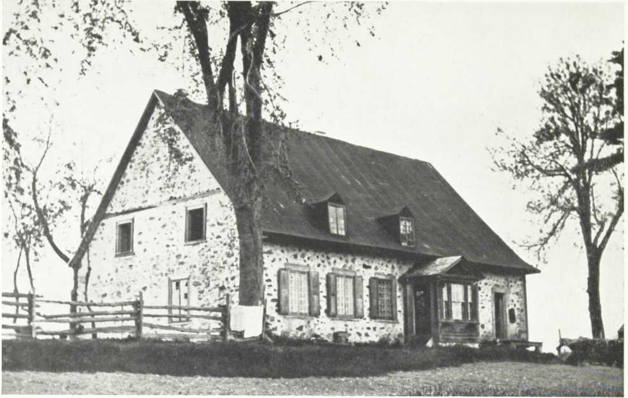
THE SOUTH SIDE BEFORE RESTORATION
