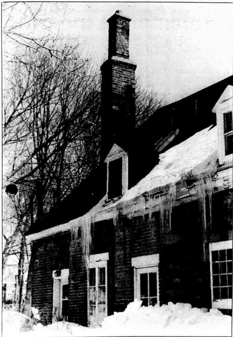
This rear view shot of the Hurtubise House annex features the chimney slated for demolition.
