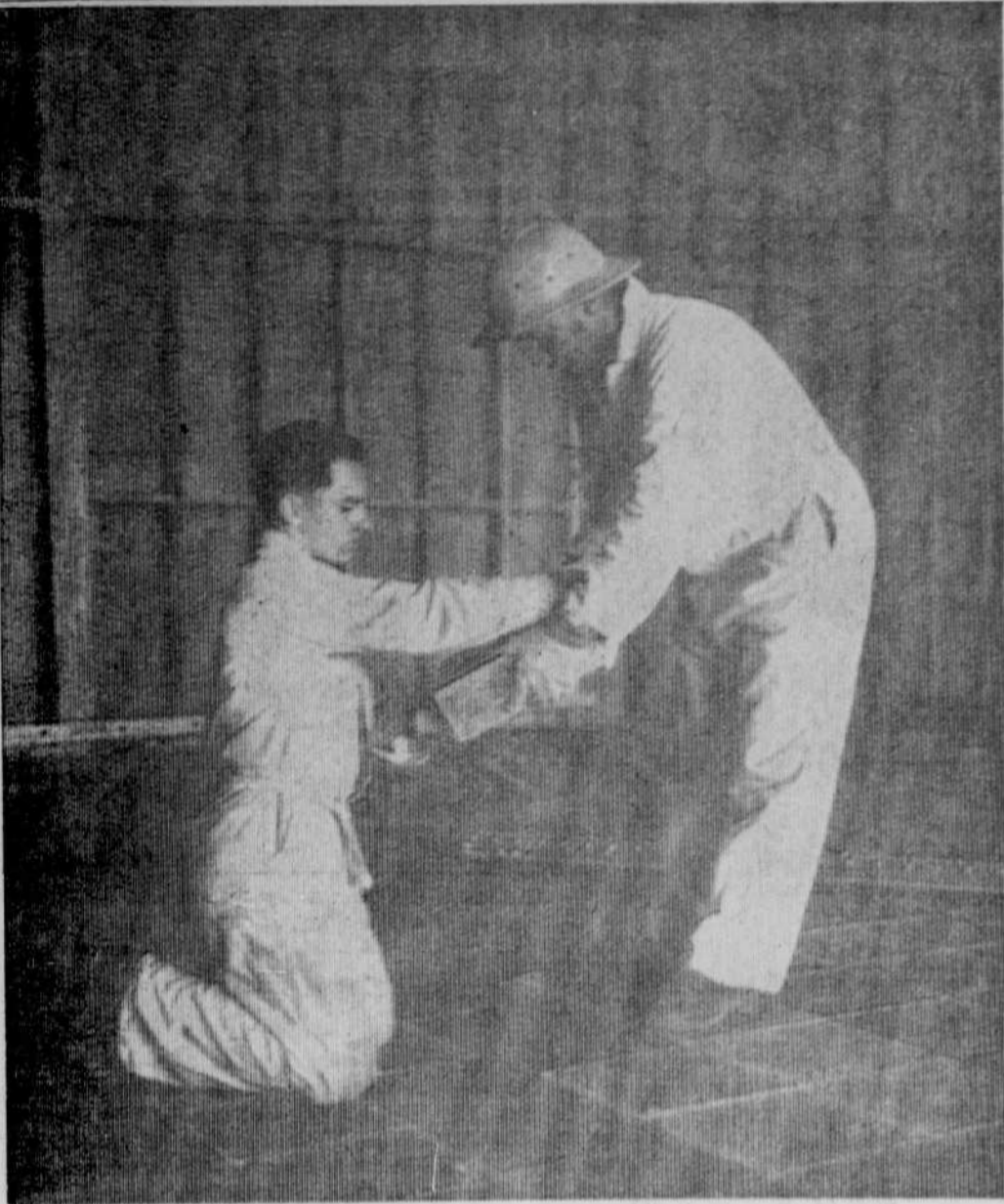
PLACING CHARGE — Two temporary employees of Sufield Experimental Station, 25 miles northwest of Medicine Hat, Alberta, are helping to build up a charge of 500 tons of TNT to be exploded tomorrow. The partially built charge they are standing on contains about 200 tons of TNT blocks. (Dept. of National Defence photo)
