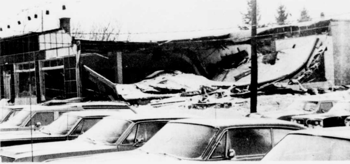
COLLAPSES AT MAGOG — The former Western Tire Store building at Magog fell prey to recent heavy snows, and collapsed, as shown in the above picture. No one was
