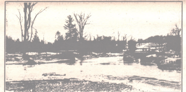
Lorimer Bridge Carried Away by Ice Jam
