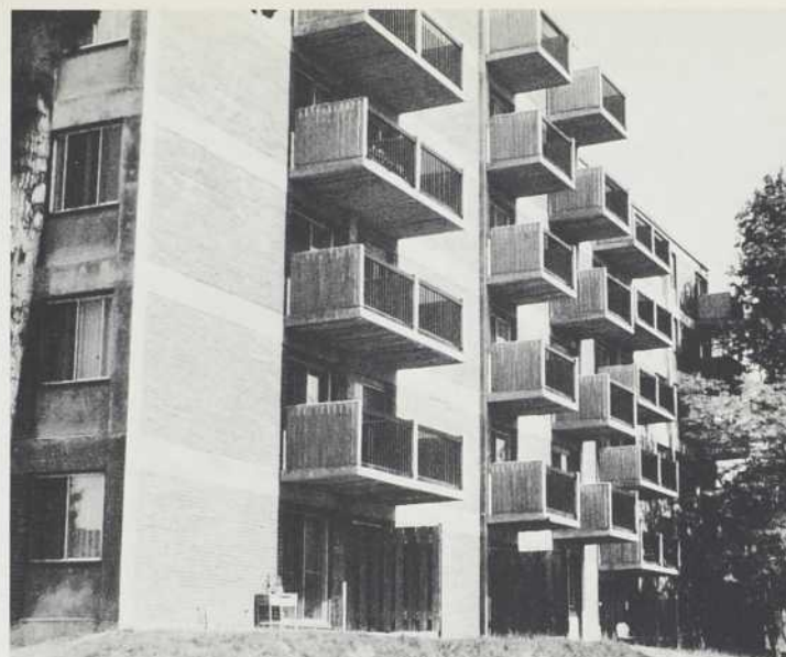
Habitations Dublin Fortune. Architecte: Jean-Louis Lalonde
