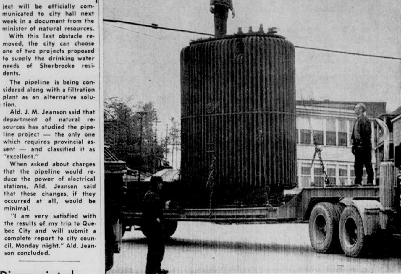
TRANSFORMERS AWAY — sub-station, being demolished, to a new home on Roy Street, near the Magog River. Being moved in this photograph is one of the city's giant electrical transformers. (Record photo by Gerry Lemay)
