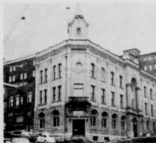
Tudor Apartments located at the corner of Frontenac and Marquette.
