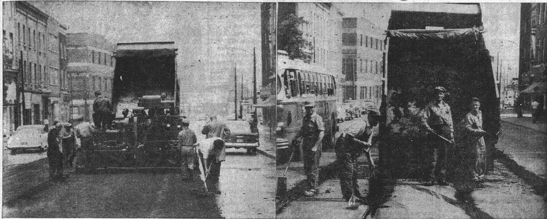
CITY WORKS department employees are rushing the repaving task on Westmount main arteries, and as these camera shots show, are covering tram-tracks, then resurfacing thoroughfares at a rapid rate, despite the July-August high temperatures. —Acme-Harrison Photo
