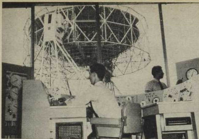
A VIEW FROM THE CONTROLLER'S DESK, IN THE CONTROL ROOM.
