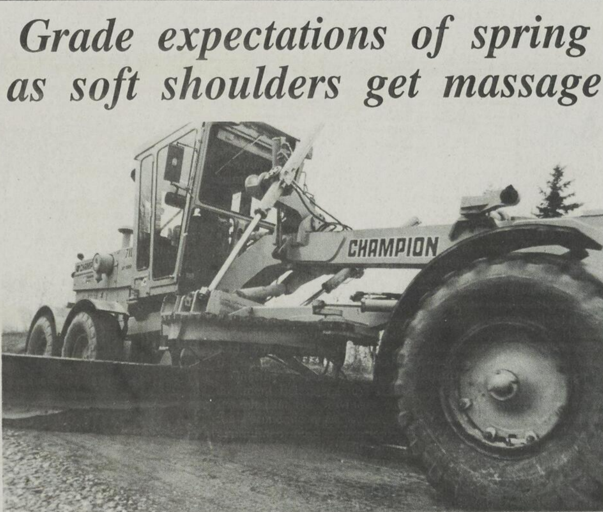
Called maintainers in our photographer's youth and graders in more modern days, these huge machines have been out in fleets around the Eastern Townships. These two were busy working with a dumptruck, firming up the soft shoulder near Sand Hill.
