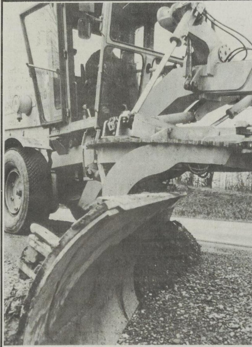
Called maintainers in our photographer's youth and graders in more modern days, these huge machines have been out in fleets around the Eastern Townships. These two were busy working with a dumptruck, firming up the soft shoulder near Sand Hill.
