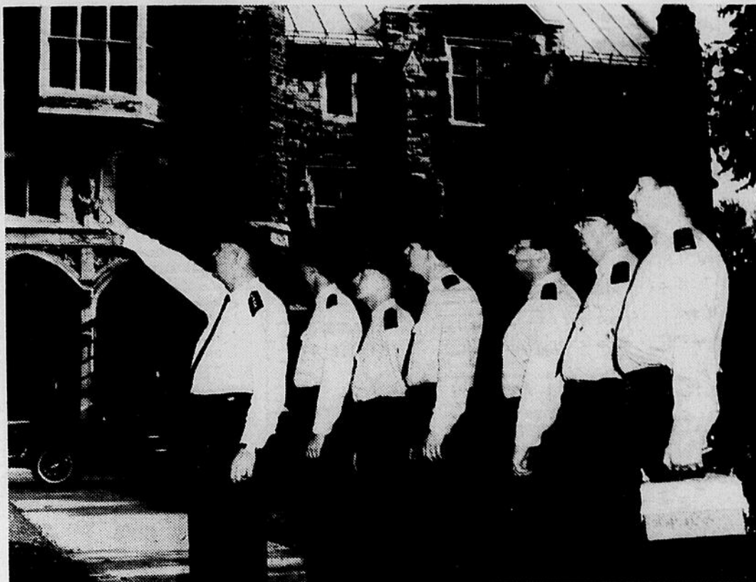
INSPECTION: Proved only this week, that building inspection pays off (fire at the Chateau Maisonneuve, Claremont and Western avenues) our fire officials get a good look at Victoria Hall. "We take special care with these older
